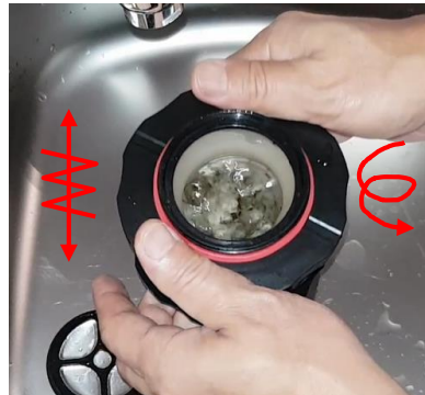
Slow pump and swirl action brings residual to bottom
